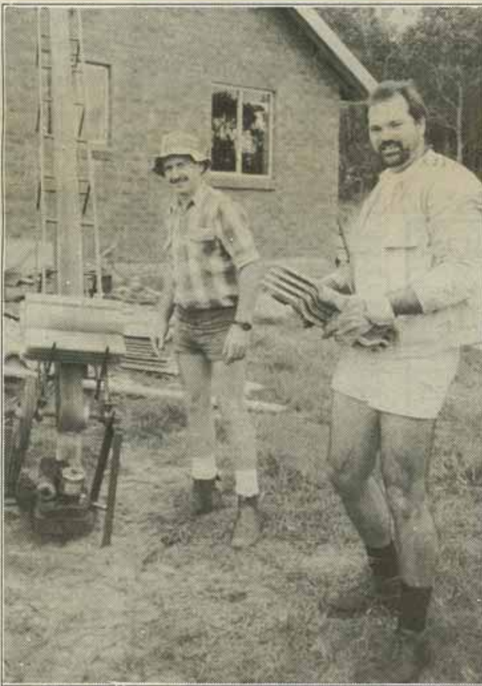
President of Jamberoo Apex Club, Allan Chittick and South Coast District Governor, John Carter load the elevators with the tiles donated by Monier Roof Tiles of Gerringong to the project.
